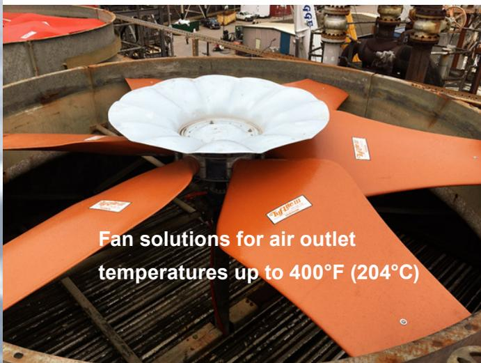
Fan solutions for air outlet temperatures up to 400°F (204°C)
